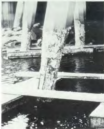
Above: Detoriated pilings can be given new life with nylon fabric forms for concrete. Right: Pilings being restored with Fabriform pile jackets. Mortar is injected through two hoses extending to bottom of jacket.
