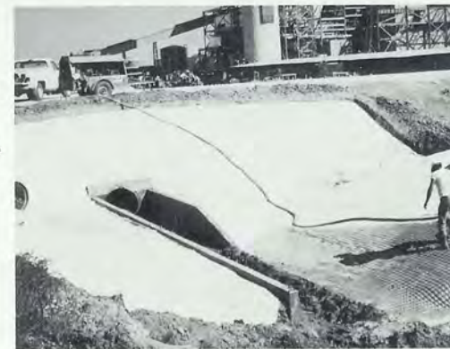
Above: Fabric being positioned along canal bank prior to the pumping of concrete. Below: Concrete being pumped into fabric form at a lake adjacent to a power plant.
