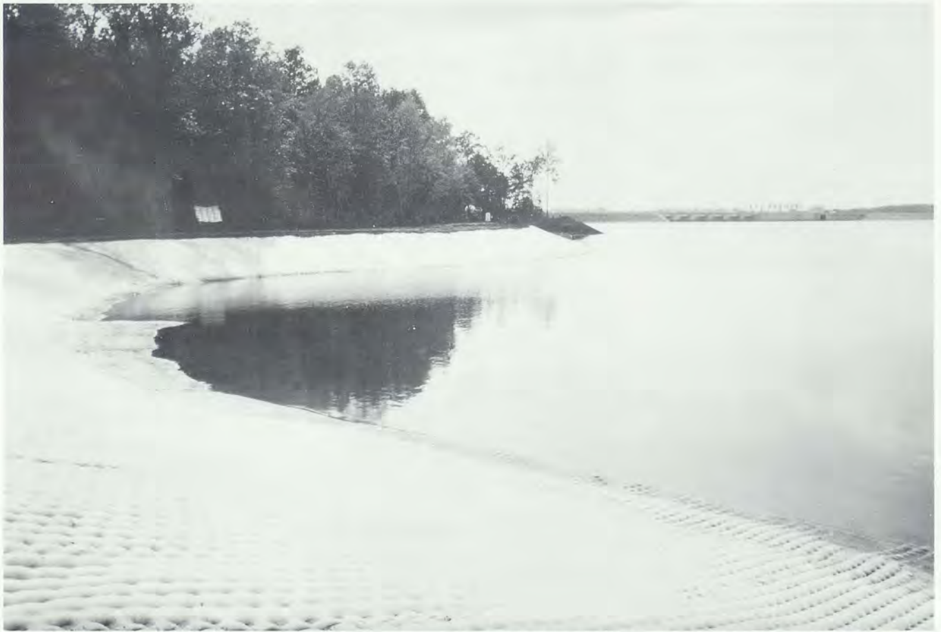
A section of the shoreline of West Point Lake in Georgia is protected from erosion with fabric concrete revetments.
