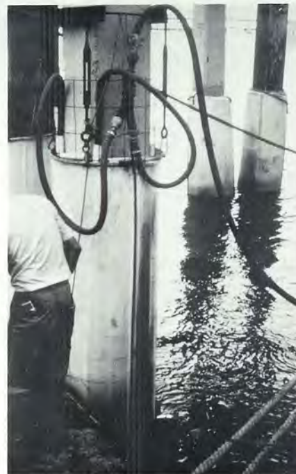
Above: Detoriated pilings can be given new life with nylon fabric forms for concrete. Right: Pilings being restored with Fabriform pile jackets. Mortar is injected through two hoses extending to bottom of jacket.
