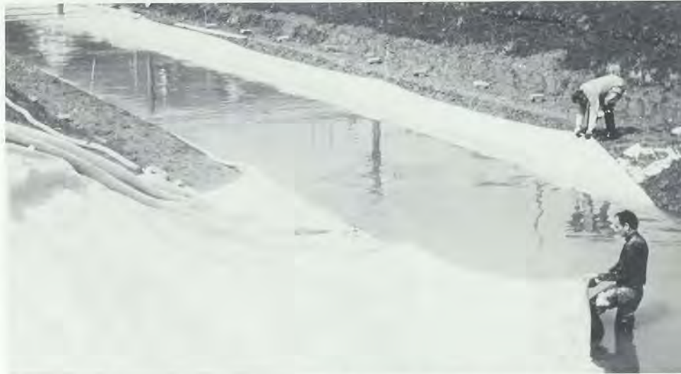
Above: Fabric being positioned along canal bank prior to the pumping of concrete. Below: Concrete being pumped into fabric form at a lake adjacent to a power plant.
