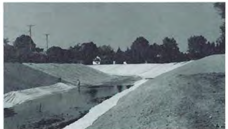
Final Fabriform work underway at the upstream end of the project.
