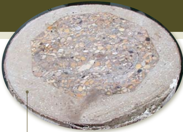
Above: Cutaway view showing the original cement pile (inner octagon) and the new Fabriform concrete pile (outer circle).
